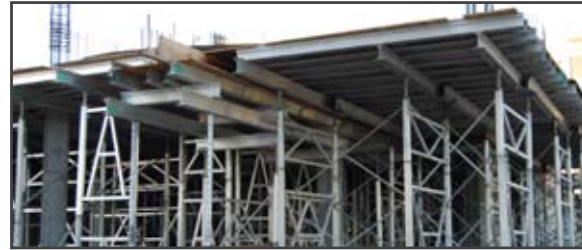
SITE CAST IN PLACE
