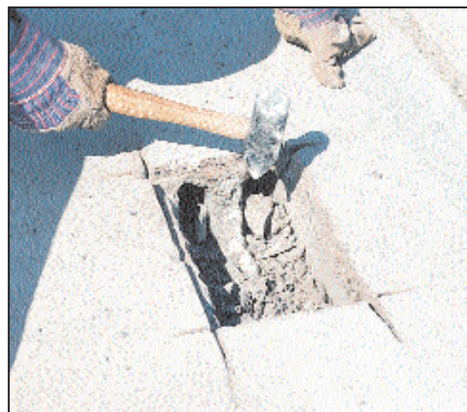
3. Break out remaining concrete with a mall.
