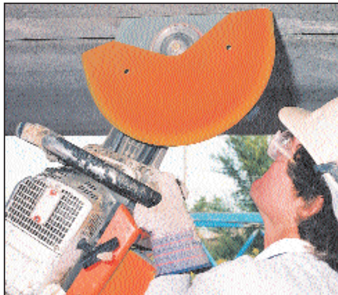
1. Cut around perimeter of opening from below.
